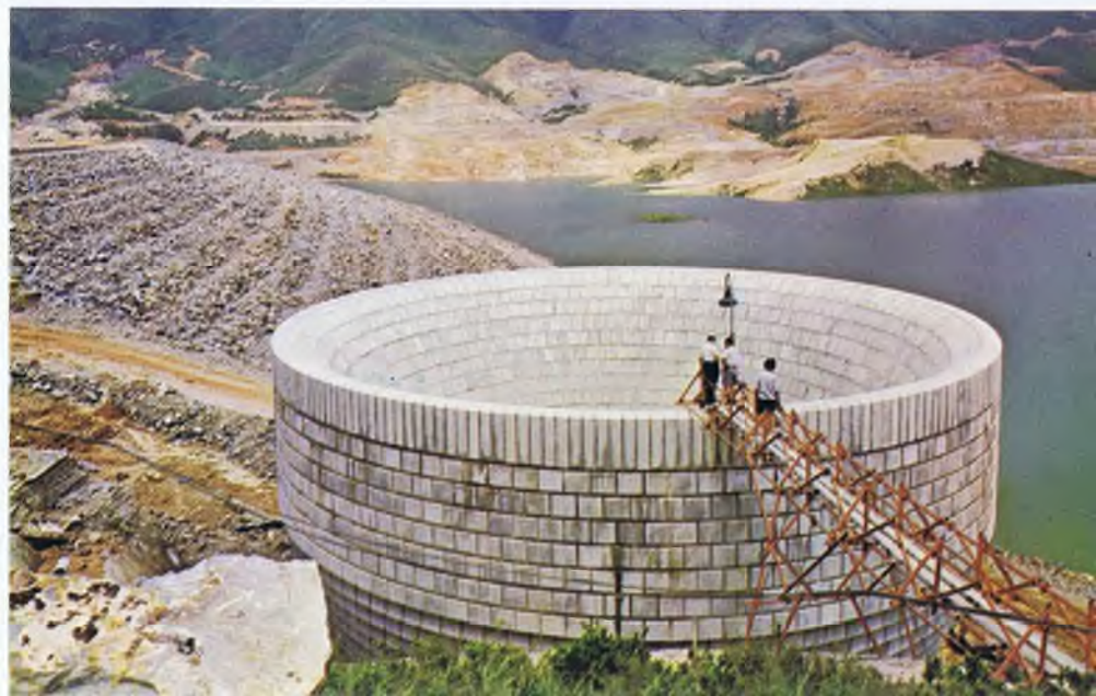
Above: The pumping station which can be remotely controlled from the treatment works. Below: The bellmouth spillway with a top diameter of 80 ft. and a depth of 165½ ft.
