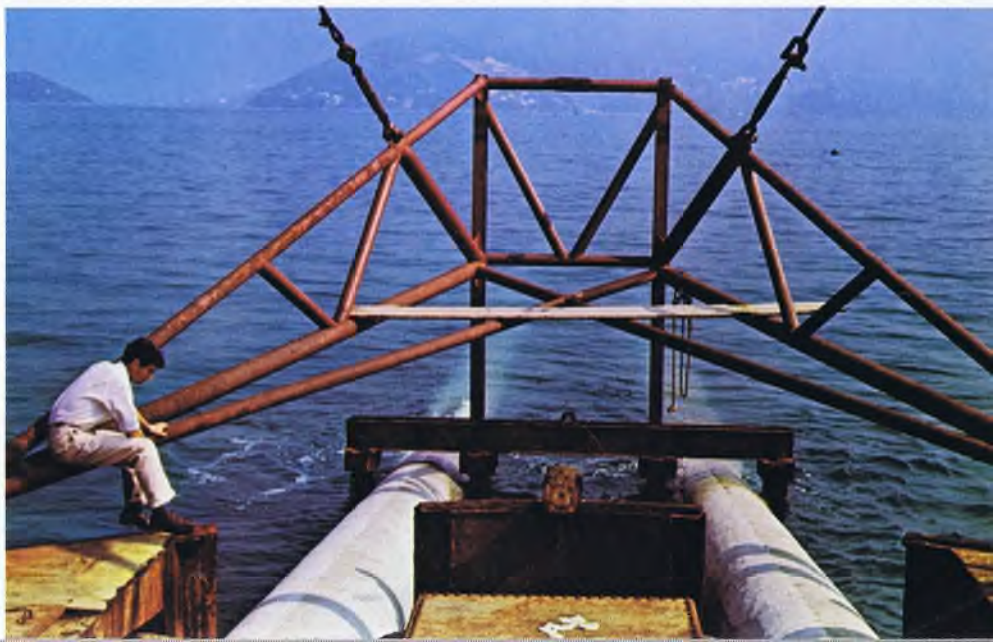
Above: A section of one of the catchwaters which feed into the dam. Below: Laying the eight-mile long twin submarine pipe-line between Lantau Island and Hong Kong Island.
