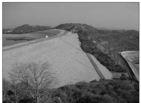
Fig. 10. Mangla intake dam
