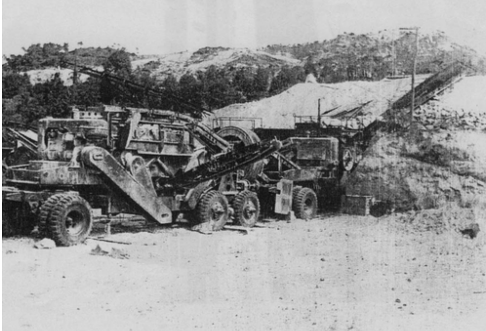
American I.O.W.A mobile crushing and screening units in the quarry
