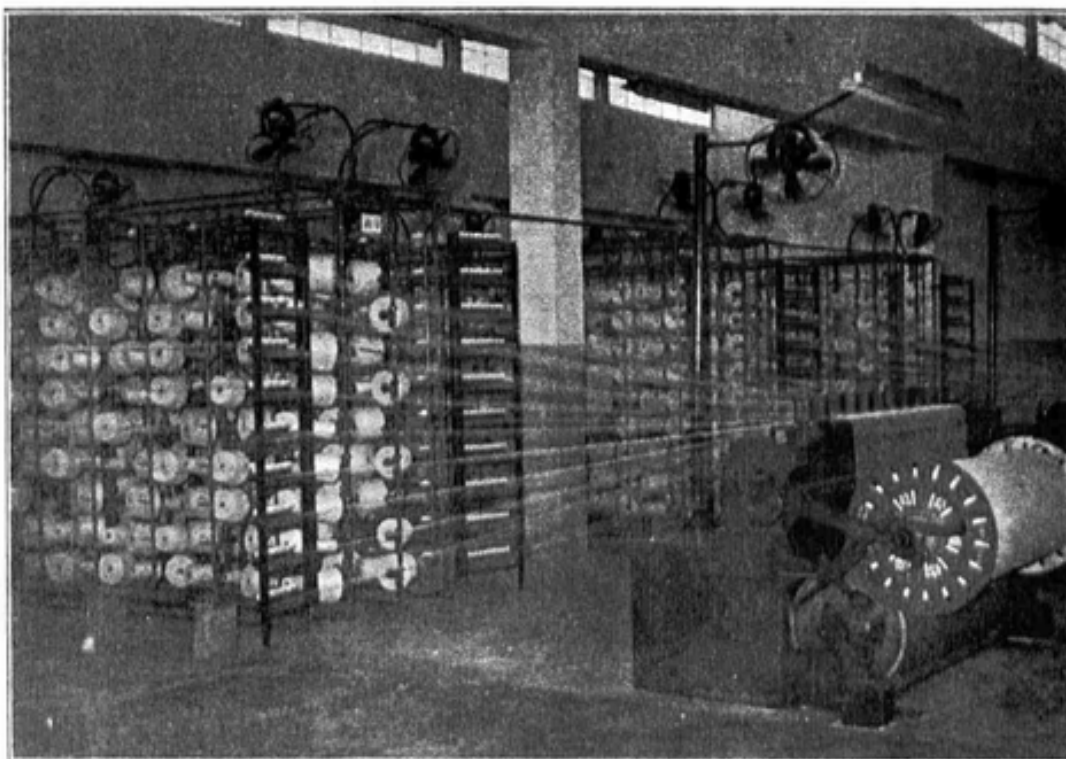
Courtesy: South China Textile, Ltd. Rapid winding on a Warpers Beam.
